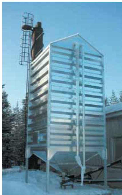
30 m 3 vertical steel silo
