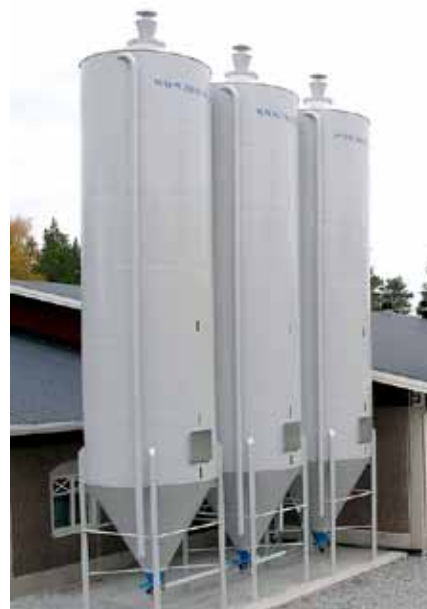
3 x 34 m 3 vertical steel silo
